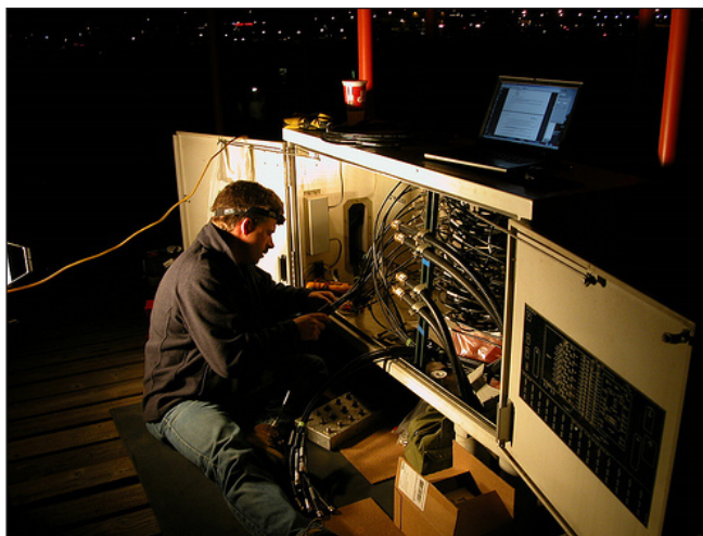
Figure 10. This system installation is configured with solid outer conductor cables. Maintenance activities are usually scheduled to avoid peak operational periods.
