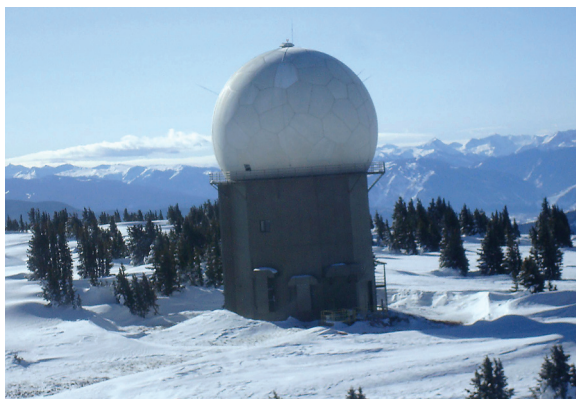
FAA Radar Station at 12,000 feet, Red Table Mountain, Colorado.
