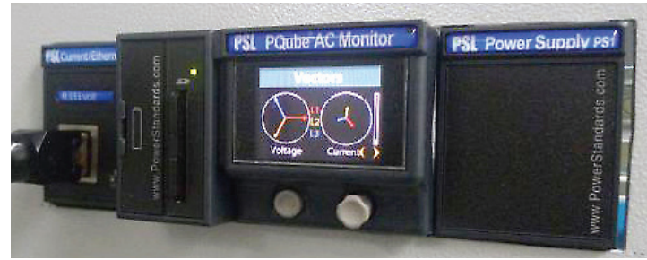
A typical PQube installation: PQube unit (middle) with a power supply module (right) and a combined current/ethernet module (left).
