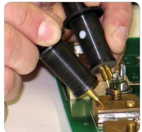
Shown here Kelvin probes used to measure contact resistance between shunt and circuit board trace
